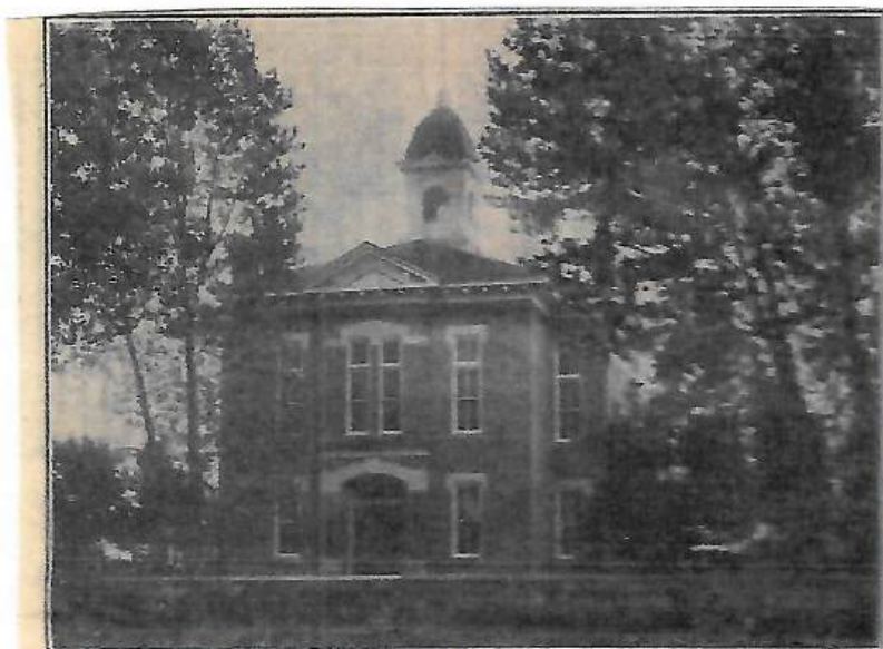
SAGUACHE COUNTY COURT HOUSE BURNED DOWN ON WEDNESDAY, MARCH 2, 1910 (Saguache Crescent, 1910)
